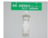
Checking office temperature and humidity on an energy patrol at the Yamanashi Plant
